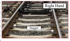
other if they are welded, otherwise short leg on curve stock rail, however 2 drawings show the stagger the other way.
